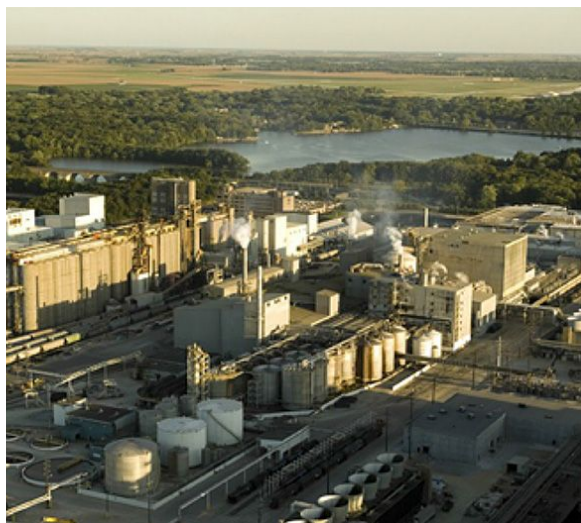
Figure 3: Archer D. Midland's Agricultural Processing and Biofuels Plant in Decatur, IL. This BECCS plant is an ethanol refinery: it ferments corn into fuel. Some CO 2 from this fermentation is being captured and stored. However, volatile organic compound emissions are high [11, 12]. (Image: US Dept of Energy)
