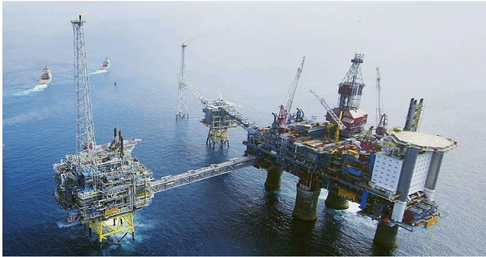
Figure 4: Sleipner Gas Field Offshore Rig, which pumps CO 2 into a deep saline aquifer. This facility has operated since 1996, and the reservoir beneath appears to be retaining nearly all of the CO 2 . [19,20]
