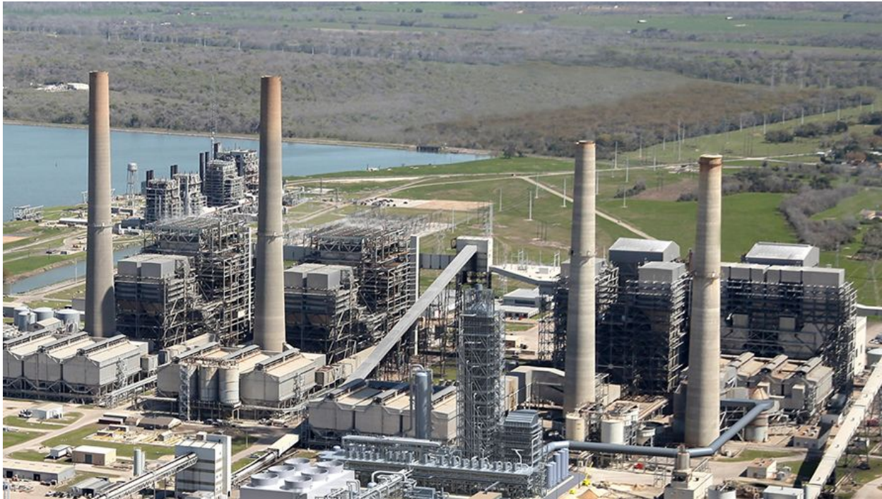
Figure 1: The Petra Nova Carbon Capture Plant, the largest in the world as of 2017 [1]. The carbon capture component of this power plant is the rectangular tower with a scaffolding of pipes in the center-foreground. This facility cost $1 billion and will prevent 0.0014 Gt (billion metric tons) of CO 2 per year from entering the atmosphere. Worldwide, about 38 Gt of CO 2 (over 27,000 times more) are emitted annually [2].
