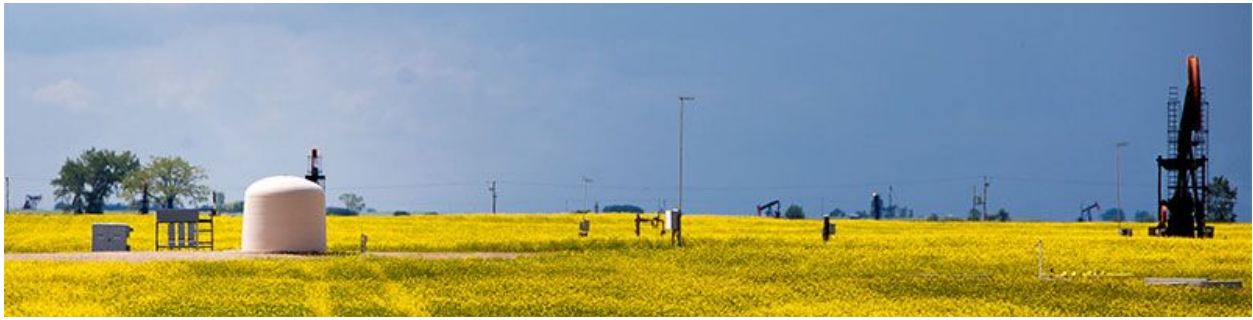
Figure 5: Weyburn-Midale Project. Observe the CO 2 injection site (left) next to an oil rig (right). Enhanced Oil Recovery has been conducted at this site in Saskatchewan, Canada since 2000. Many other oil fields in nearby Manitoba and North Dakota also use EOR. [22-23]
